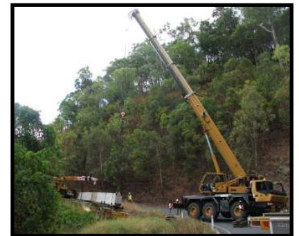
2010 Winning Category B Lift - Kelly's Crane Hire
