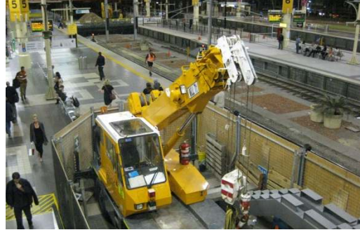
Freo Crane At Work At Perth Railway Station
