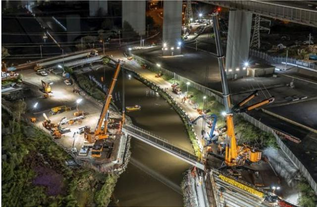
When lifting loads with cranes, concentrated outrigger pressures or track pressures can be imposed on the working platform. This in turn can lead to significant deformation of the working platform and subsequent overturning of crane. Crane accidents because of working platform failures have occurred in the past.
