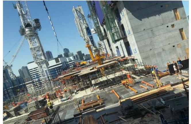
Causal Factors for the 9 ‘Crane Impacts’ were made up of 3 “Snagged loads” of which 2 were scaffolding related (1 empty hook and one tag line).
